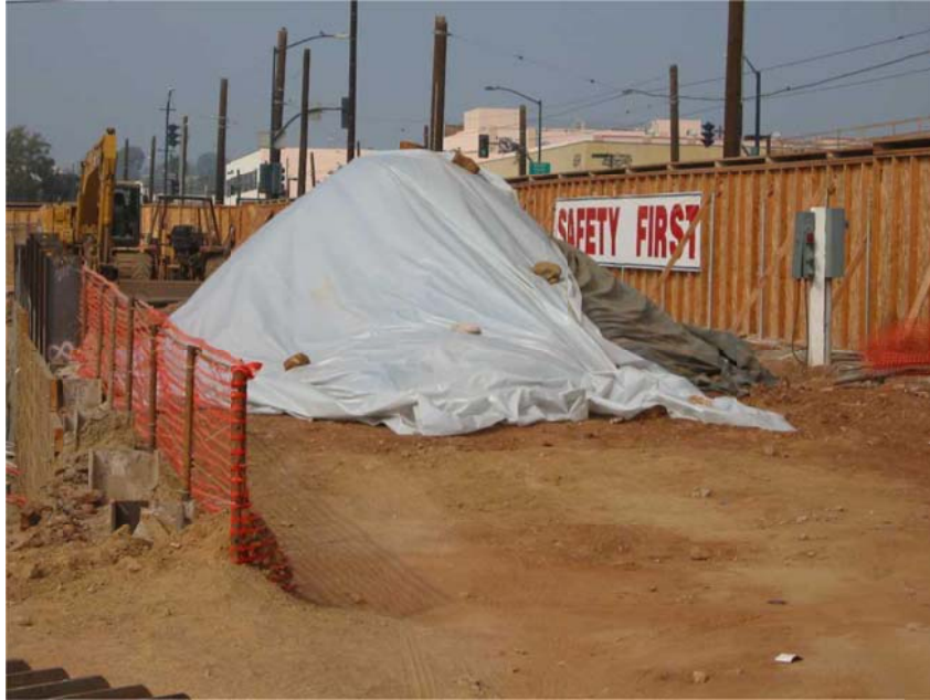
Stockpile covered with plastic and secured with large rocks.
