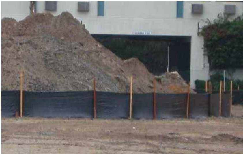
Silt fence used for stockpile perimeter control.
