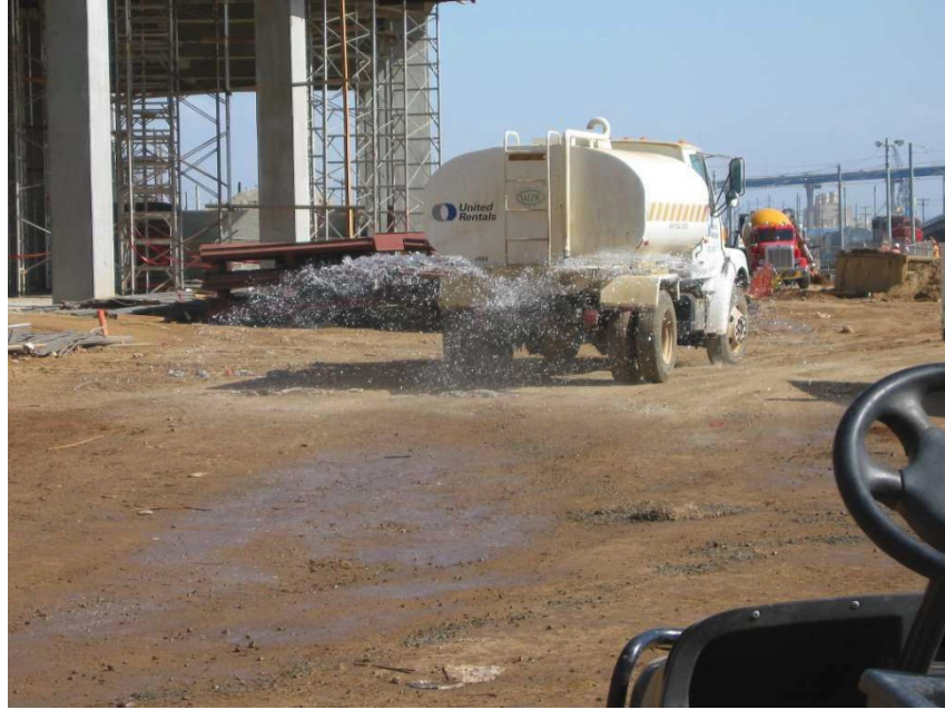
Water being applied for dust control.
